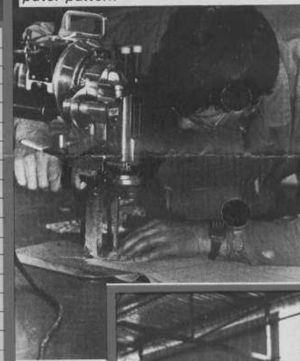
Cutting the tent membrane to a computer pattern
