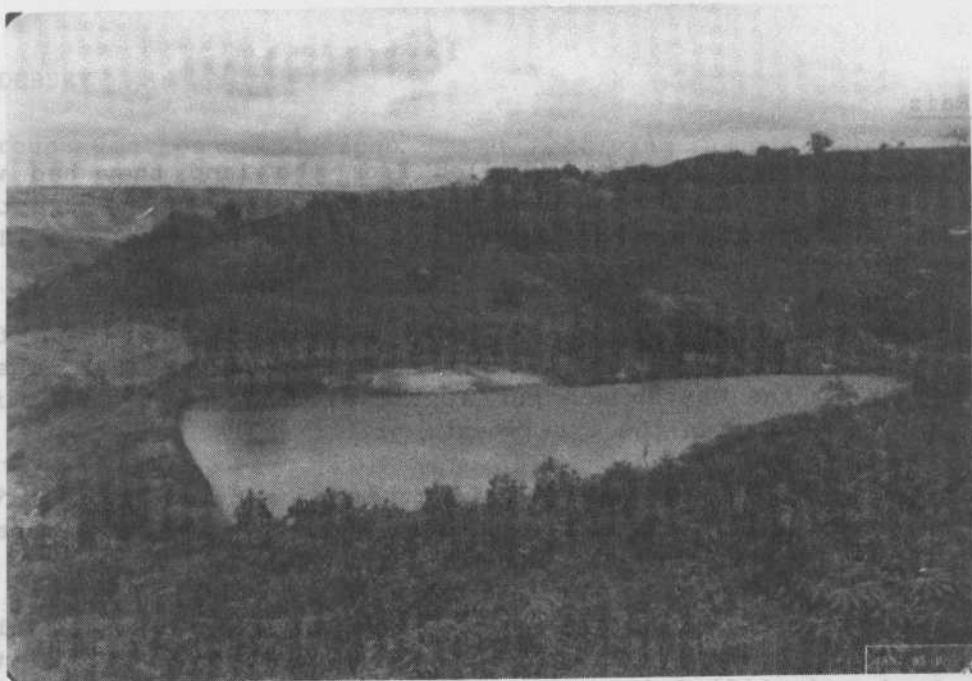
*View of dam after the rains (June 1984). Notice that the dam wall is wider. Grass was planted on it to prevent damage by rain water.*
