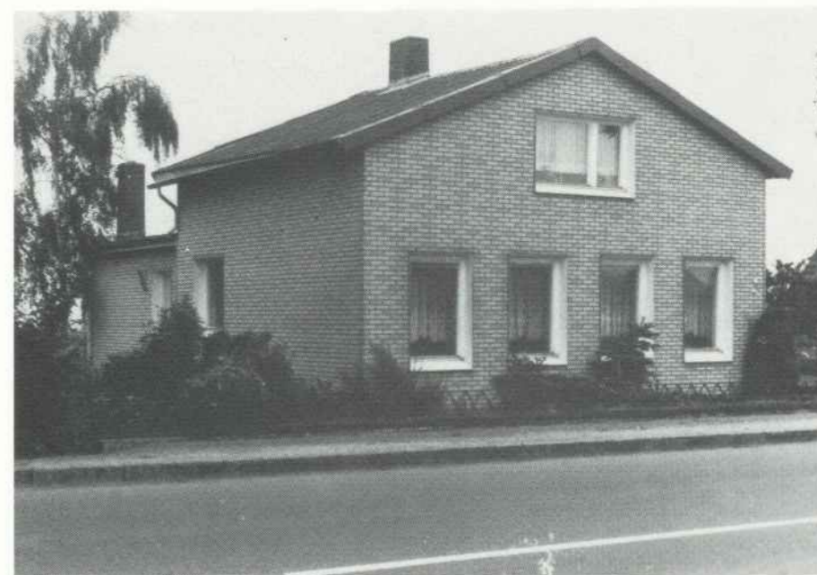
Hauptstraße Nr. 11: 1912 erbaut Martin Ahsbahs - 1953 Hans Ahsbahs - 1975 Hans Peter Ahsbahs.
